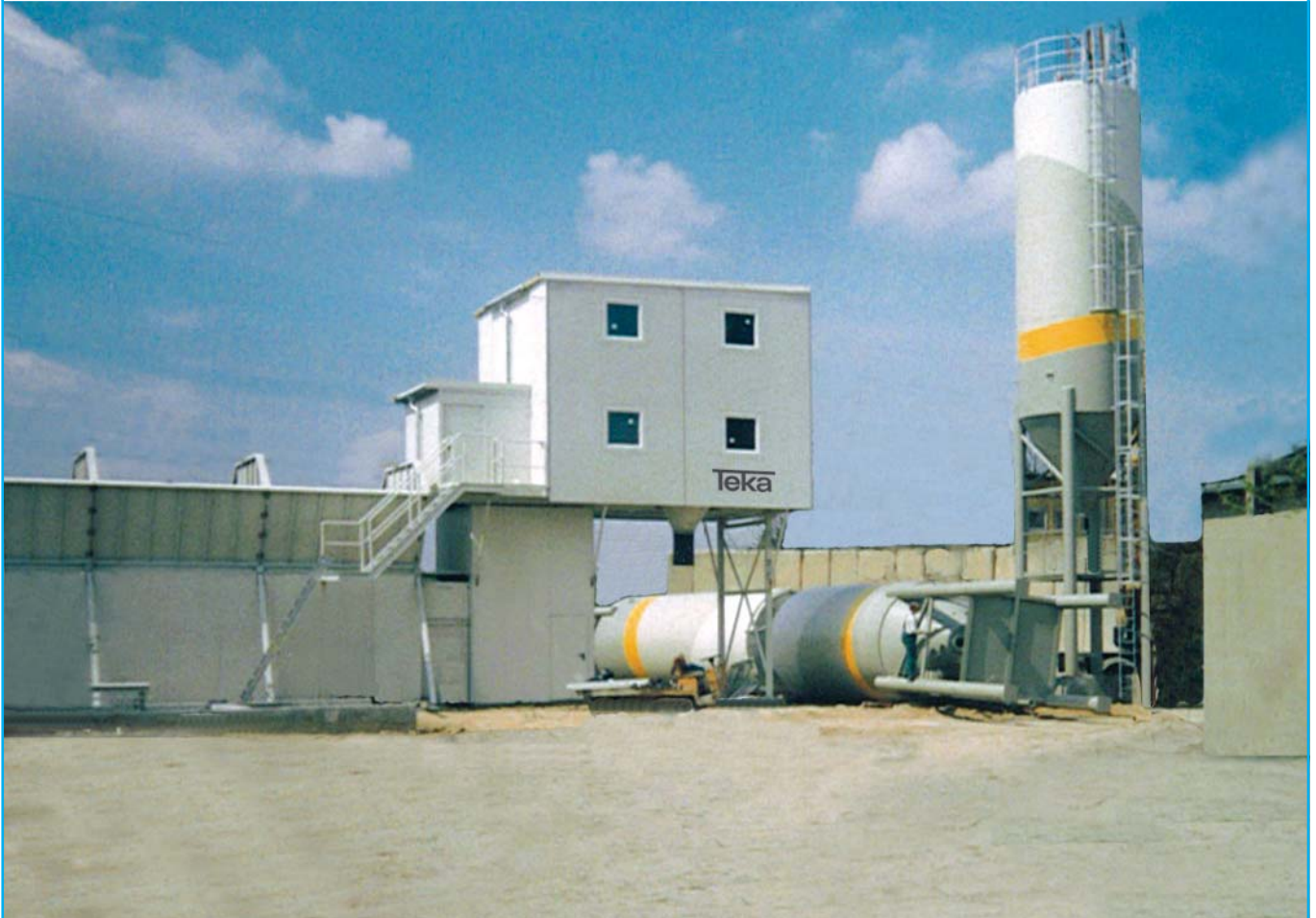
Montage MIXOMAT THZ 3000 C 1 - R • Erection MIXOMAT THZ 3000 C 1 R
